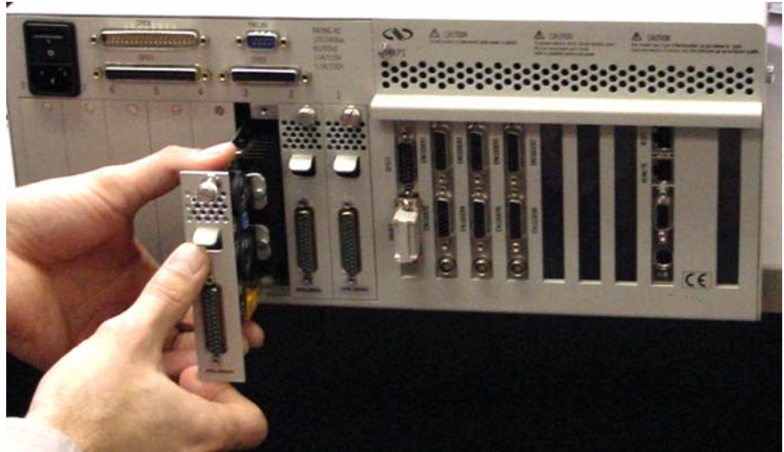
Figure 11: Installing Driver cards.
