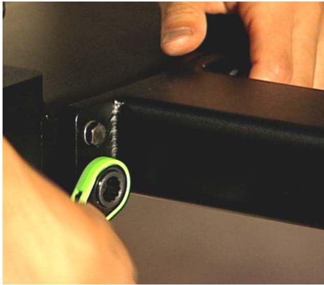
Figure 5 Tightening the cross-brace bolts to the leg weldment
